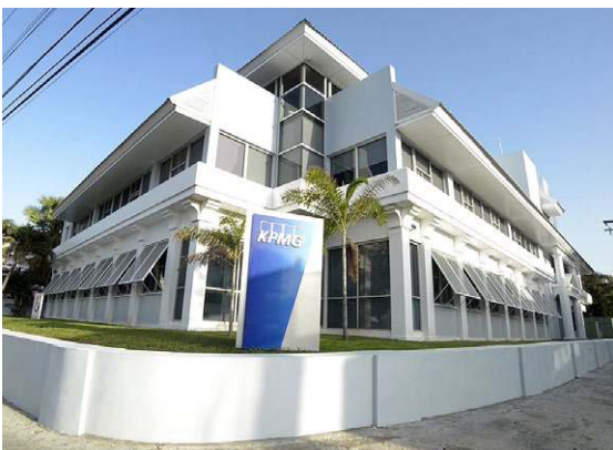
Hastings Office Centre Hastings, Barbados
