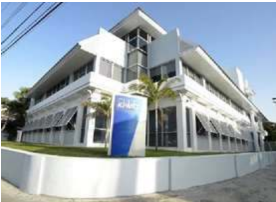
Hastings Office Centre Hastings, Barbados
